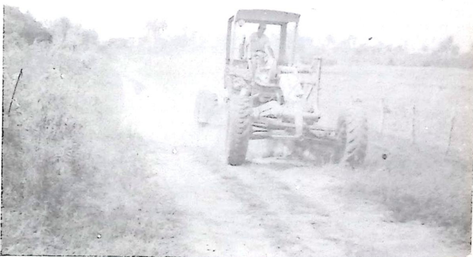
As motoniveladoras recuperam as ruas do Distrito
